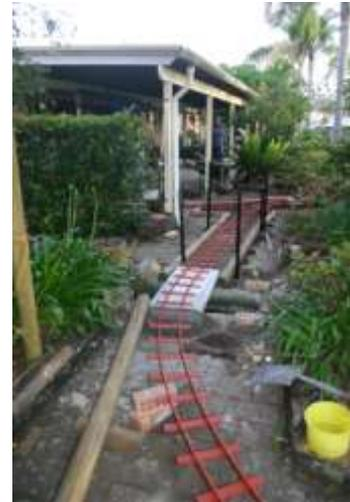
We then used bricks, pavers and blocks and a "Cowley" level to check the heights all around the track and found that if we got a bit serious with the earthworks then we could make the track itself almost flat. There would be embankments and cuttings, which are fun, and relatively little of the garden would need to be transplanted.
