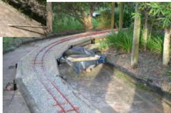
Once the track was finally joined up, joint by joint it was brought up to level and then the ballast evened out. By about 7pm the track was running!
